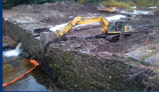
Beginning of Dam removal.
